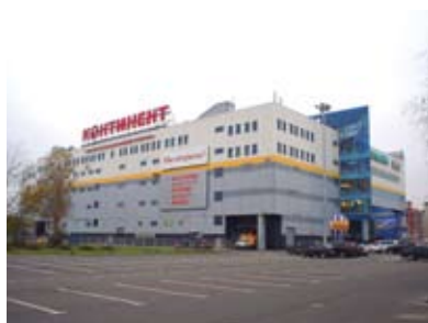
The largest shopping centre commissioned in Q3 2007. Retail-entertainment centre Kontinent-2, Baikonurskaya st., 14a
